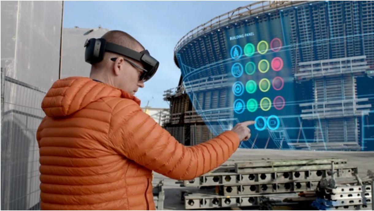
Bentley's SYNCHRO XR and Microsoft HoloLens 2 bring the benefits of mixed reality to construction sites.
